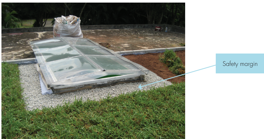
Fig 14 : The fire safety margin around a protruding skylight of a rooftop greenery. This margin must be kept clear of vegetation.
